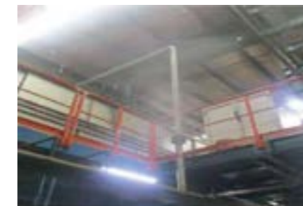
Reduce energy consumption by stopping extra running pump.
