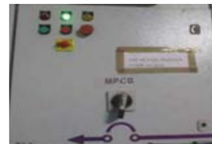
The DCC make-up pump now operates based on the DCC tank's water level switch, shutting off at high levels to save electrical energy.
