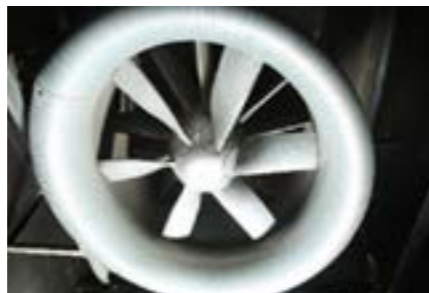
Air Handling Unit-Centrifugal blower replaced with energy efficient axial flow fan.
