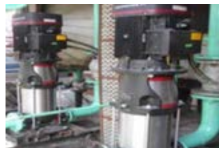
Replaced 11 old conventional pump with energy efficient pumps.
